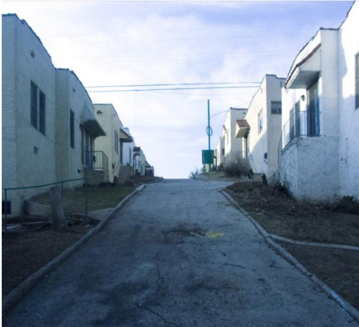
Looking west towards Maltman Avenue along central driveway just prior to construction.
