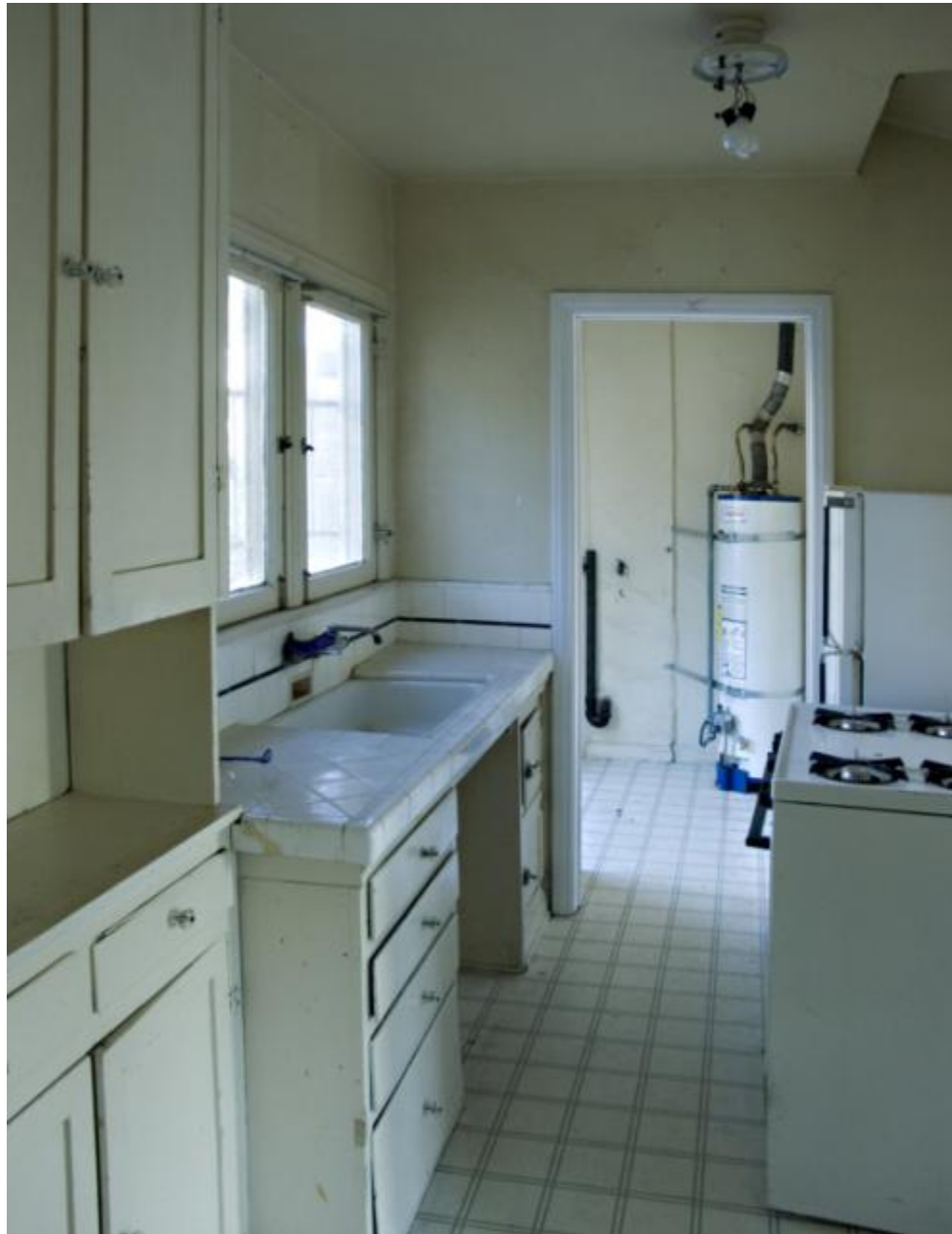
Typical kitchen and utility room prior to renovation.
