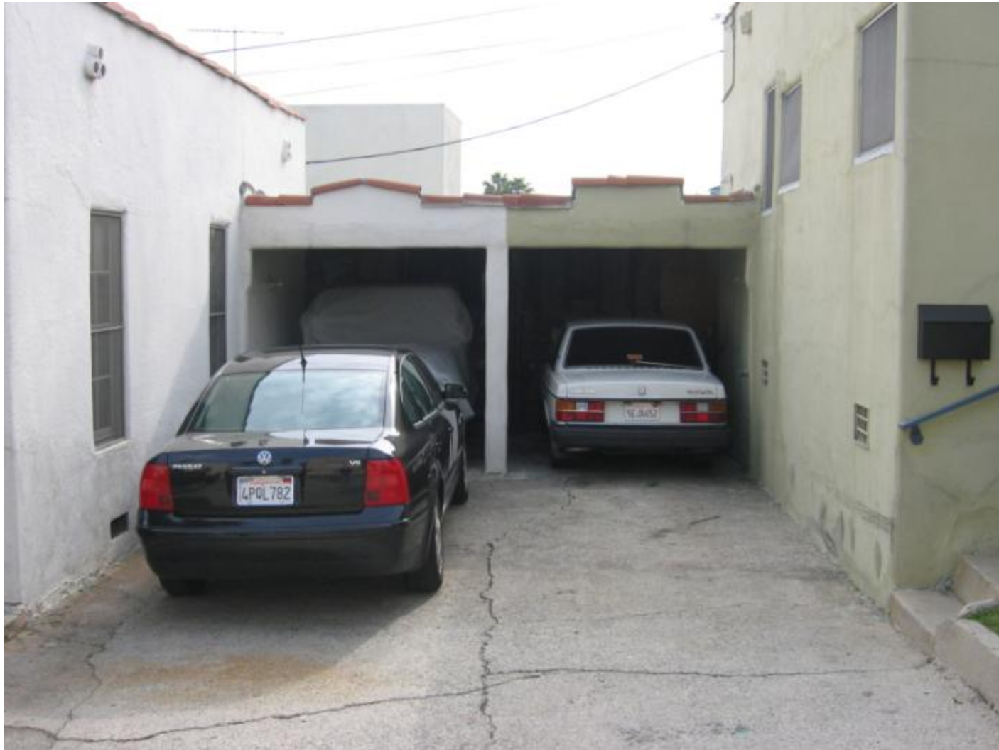
Original attached garages prior to renovation.
