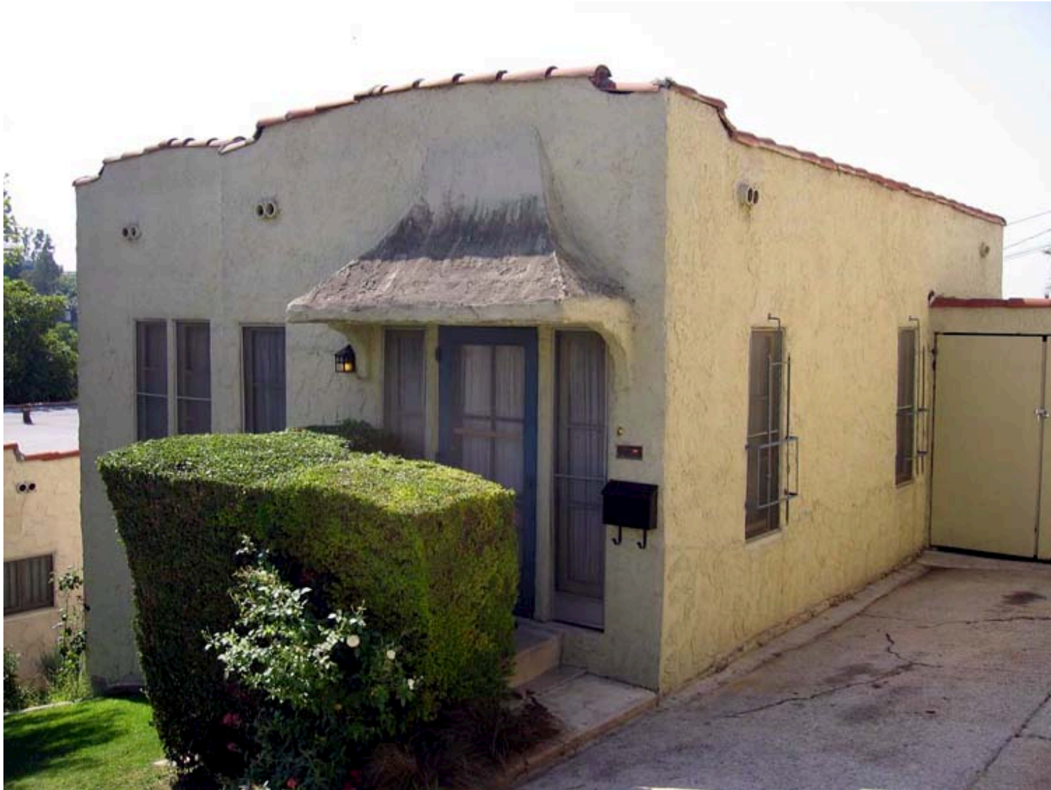
One of the bungalows prior to renovation.
