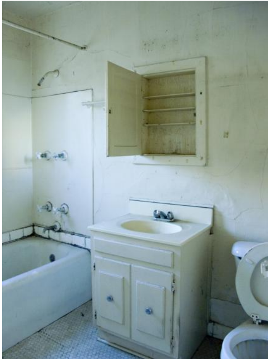
Typical bathroom prior to renovation.
